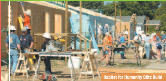
Habitat for Humanity Build
